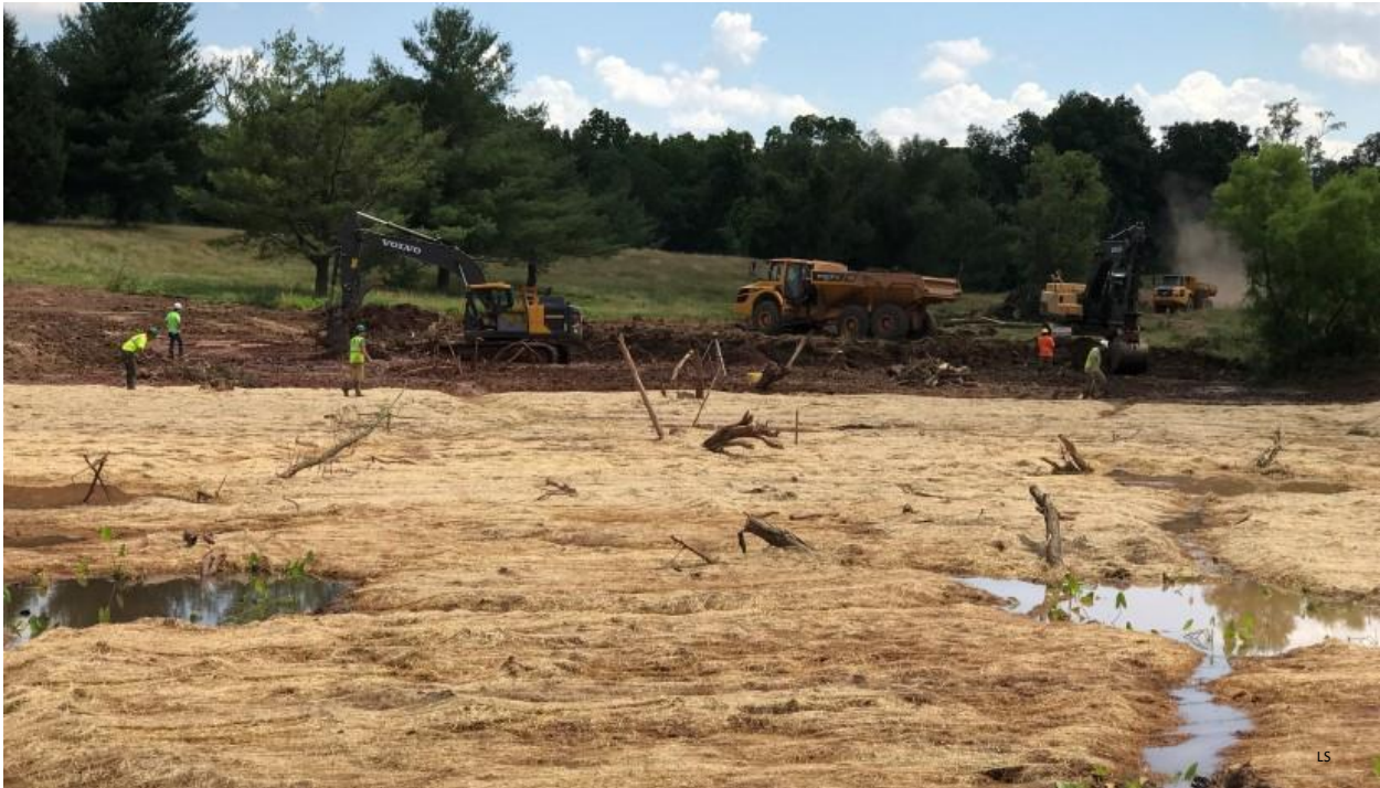
Figure 7 - Specialized contractors are used to carefully peel back the layers of sediment and expose the historical wetland.
